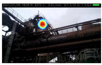
Compressed gas leak from the pipe in high place out of reach is found.
